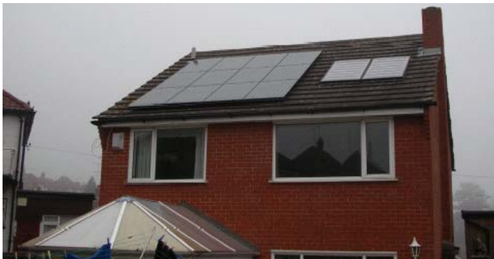
Photovoltaic PV panel (left) and flat plate solar hot water (thermal) panel (right) (source Chelsfield Solar- Entec)
