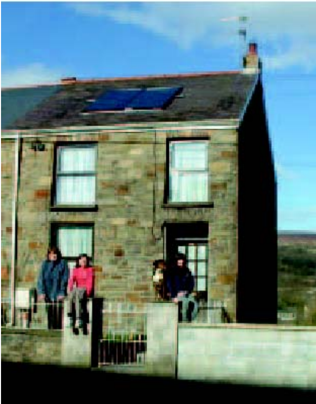
Solar thermal flat plate collectors (source Awel Aman Tawe-WAG)
