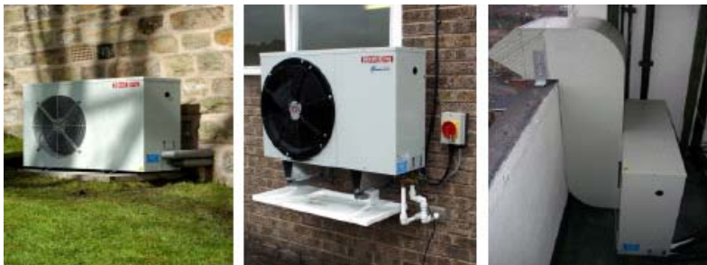
Air source heat pumps ASHP -various mountings. (source Entec)
