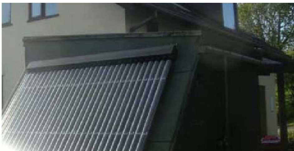
Solar thermal evacuated tube collectors sited off roof to face south (source WAG)
