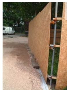
Part finished temporary surface within Root Protection Area carefully designed and supported with method statement and Arboricultural Watching brief.
