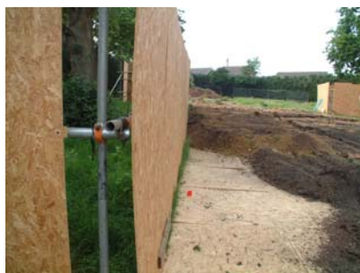
Part finished temporary surface within Root Protection Area carefully designed and supported with method statement and Arboricultural Watching brief.
